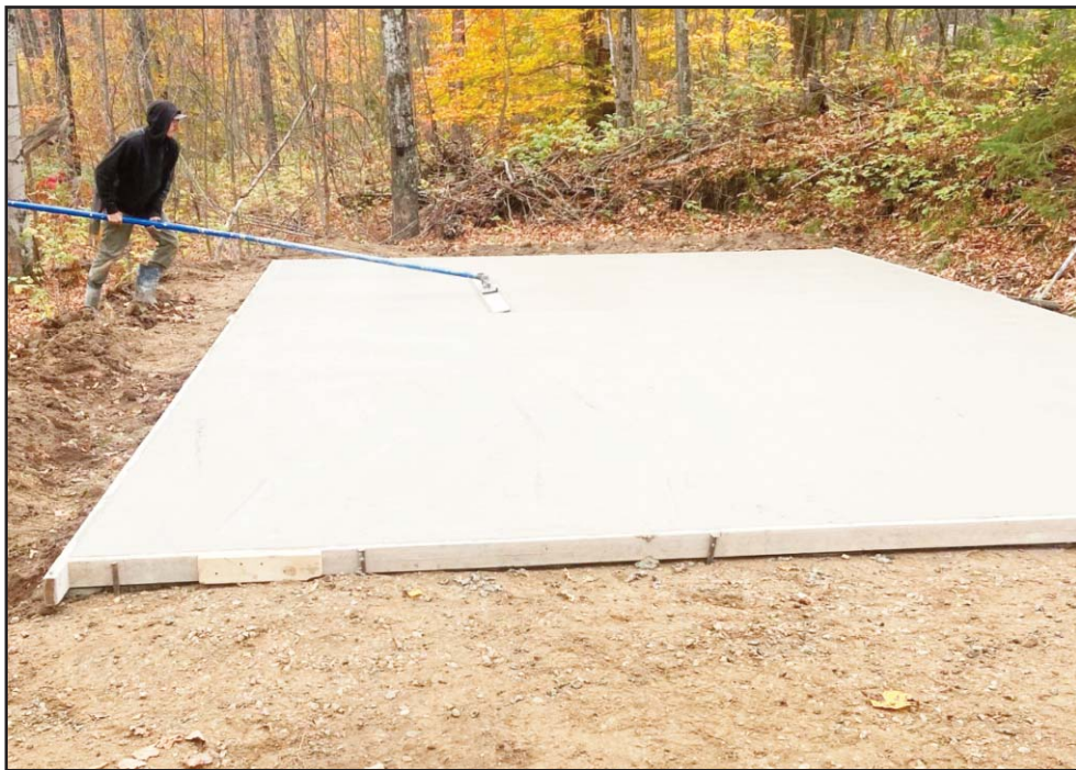
A worker smooths the freshly poured concrete slab for the Northern Lakes Archers' new pavilion. The club is raising funds for the pavilion structure, with installation planned for spring.
